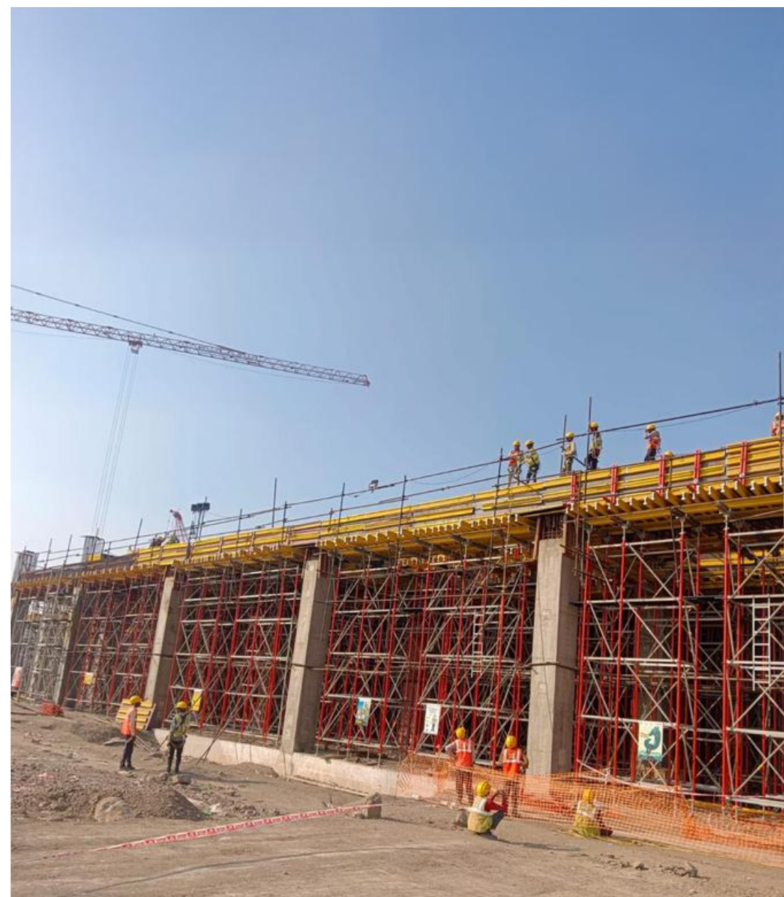
Equipment name : Peri Up MI System for Beam Bottom Country of origin : Germany Amount invested : ₹18.7 crores 1
