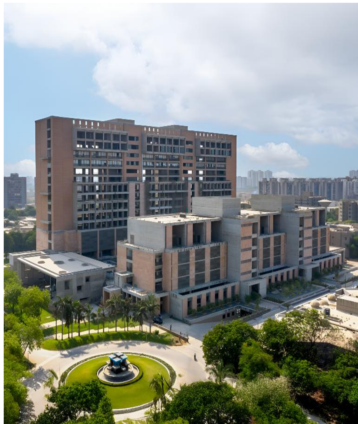
Nirma University – Old Building
